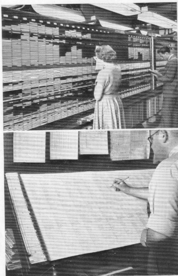
Fig. 41—Part of the shop loading chart which is really an elaboration of the pre-planning chart shown above, but records job times in detail. The chart is in the form of a continuous sheet which is wound in on a roll by the handle seen bottom left.
